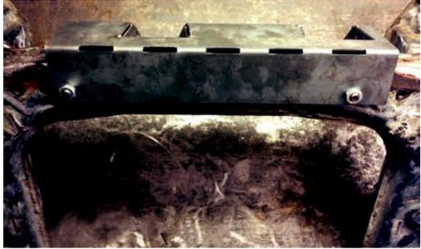
Using the template mark the holes of the cut outs and clearance holes underneath.
